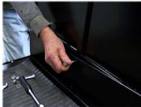
Bolt Handrail to Platform.
