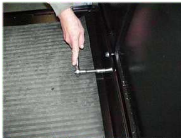
Bolt Handrail to Platform.
