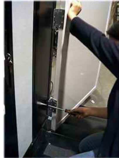
Mount the Carriage Gate.
