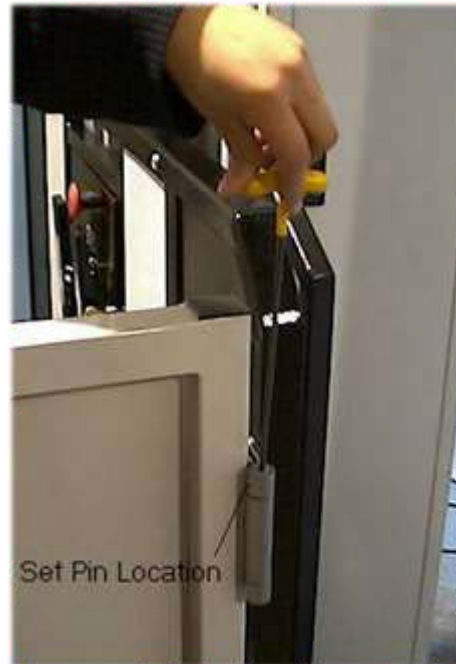
Adjust the Spring Loaded Hinge.
