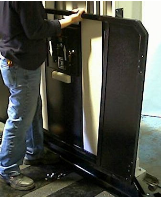
FIG. 5A- INSTALLING CONTROL WALL EXTENSION
