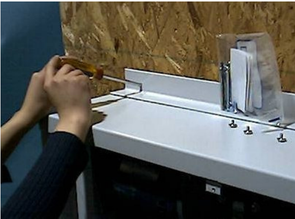
FIG. 22- MOUNT TOWER TO EXISTING STRUCTURE
