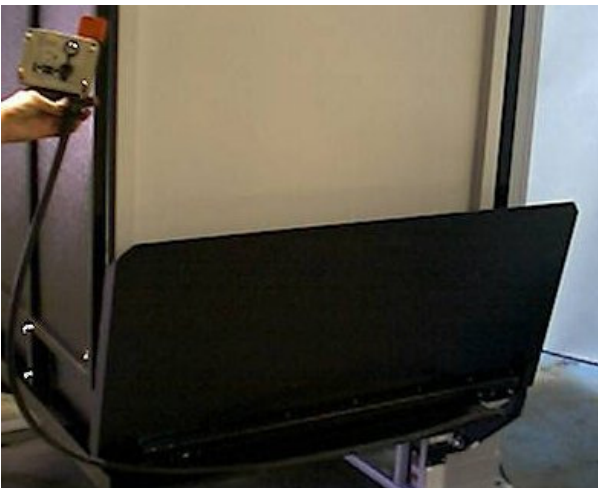
FIG. 10- RUN CABLE UNDER TOE PLATE
