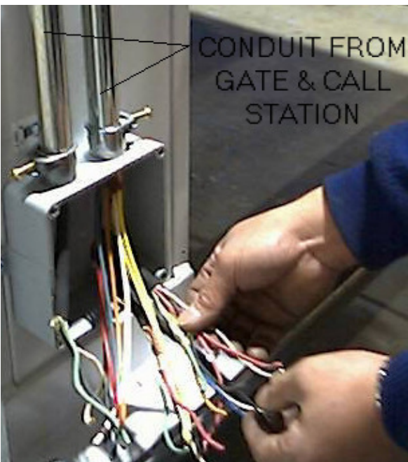
FIG. 18- WIRING OUTSIDE JUNCTION BOX
