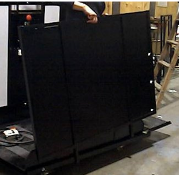
FIG. 6A- LOWER THE HANDRAIL INTO PLACE
