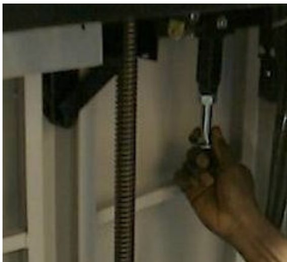
FIG. 20- INSTALLING MECHANICAL STOPS
