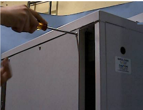
FIG. 23- INSTALL FRONT PANEL
