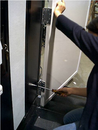
FIG. 8- MOUNTING GATE TO CONTROL WALL EXTENSION
